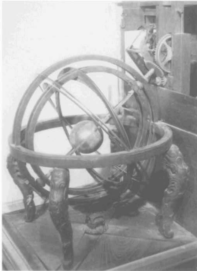
FIG. 10.6. THE KORYŎ UNIVERSITY SŎN'GI OKHYŎNG (DEMONSTRATIONAL ARMILLARY SPHERE). Believed by Needham and others to be the Sŏn'gi okhyŏng described in Korean records as having been made in 1669 and repaired and copied during the eighteenth century, but argued here to be of the second half of the eighteenth century. The armillary ring assembly is shown. In addition to a fixed terrestrial component, consisting of the outer horizontal ring with intersecting meridian (double) and equator (single) rings, there were clock-driven rotating solar, sidereal, and moon-path components, although the solar component is now missing. (For the terrestrial globe, see figs. 10.8 and 10.9.)
